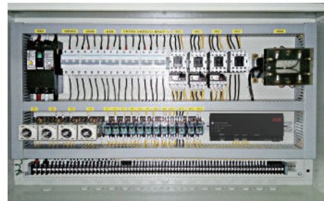
Power control cabinet
